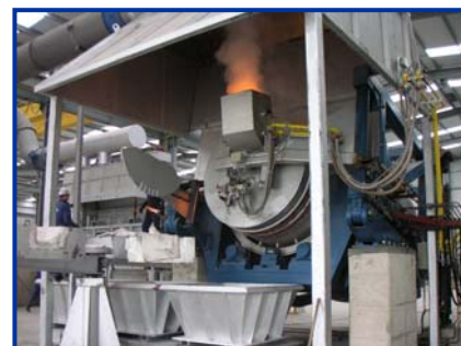
Rotary FARB Installation
