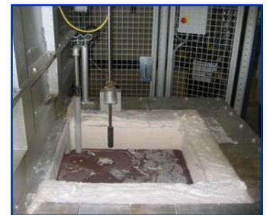
Side Well detail, Thermocouple and molten metal level sensor
