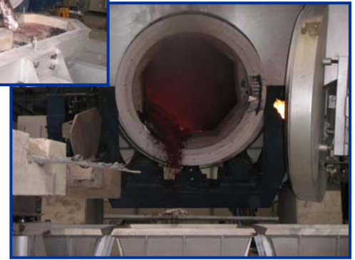
FARB with door opened, drain off molten metal with dross rake and saltcake into bins of Salt car
