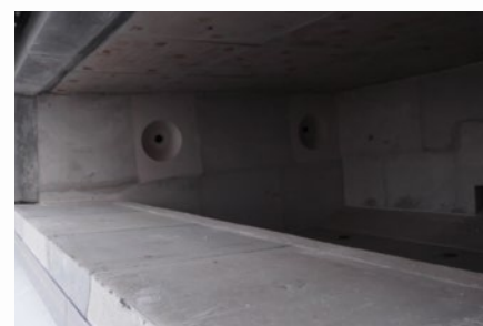
\ Precast shape on dry hearth
