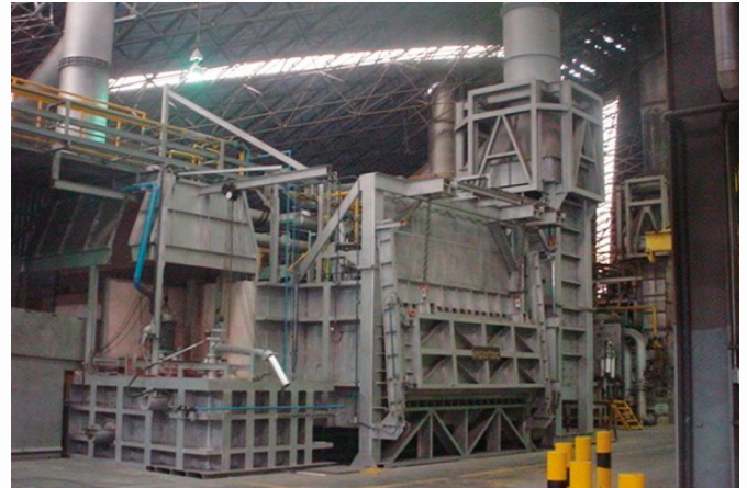
\ Stationary Sidwell Furnace 70 Ton capacity & 8 Ton/hr melting rate.
